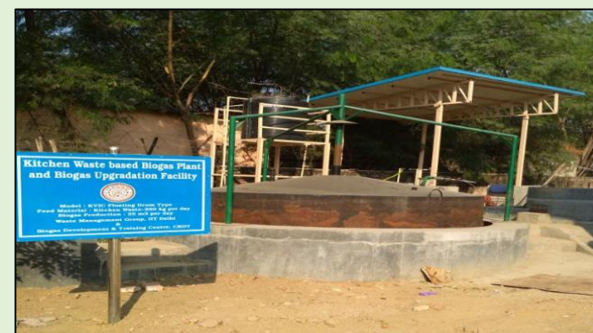
Kitchen waste biogas plant at Biogas Research Laboratory, Micromodel Complex, IIT Delhi
