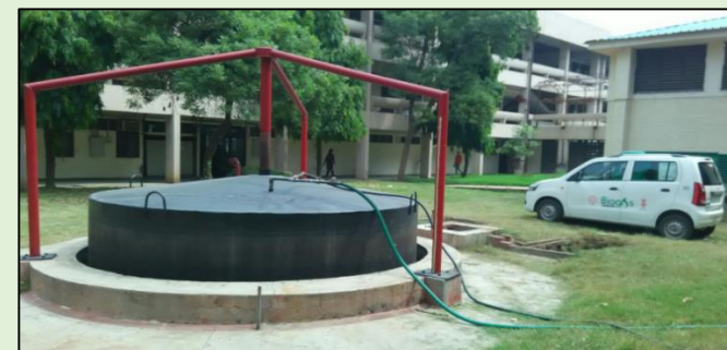
Biogas Production, Enrichment & Bottling Laboratory at IIT Delhi
